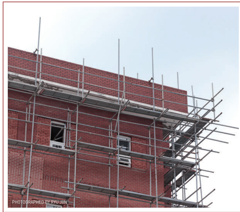
| A Modern Construction Near an Antique Temple
